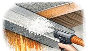
Spray-on fireproofing materials
